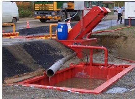
With an additional, external recycling tank to improve the water recycling.
